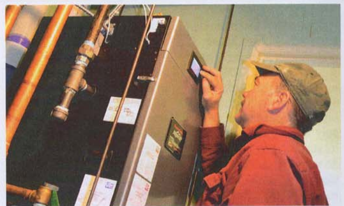
(above) Scott Seib, owner of Seib Plumbing & Heating, checks runtime hours on a 285 MBH Burnham Alpine boiler. (below) Oversized connected load, a wide variety of room sizes, and leaky pipes made the Arcadia Hall project a challenging steam-to-water conversion.
